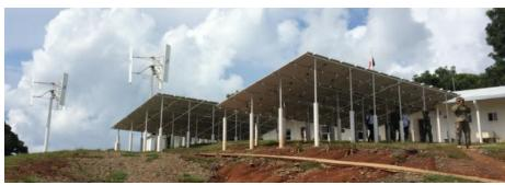
At Punto Coco, Panama, HCS Group designed a hybrid solar/wind power system for the Counter Narcotics Forward Operations Base. The system was designed as a Resilient Islanded Micro-Grid network providing primary power with banks of battery supplies to store enough energy to supply the base with sufficient power for running 24/7 mission
