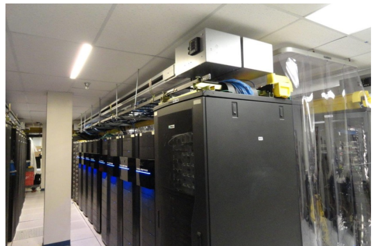
Electrical Data Room Upgrade Walter Reed National Medical Center Bethesda, Maryland
